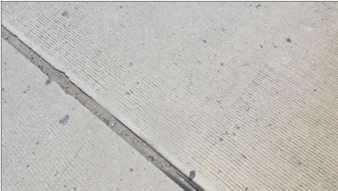
THERE ARE SEVERAL H/L CRACKS EMANATING FROM JOINTS 1' TO 4' INTO THE SPANS IN ALL SPANS. DECK HAS FEW TRANSVERSE CRACKS IN THE ROADWAY SURFACE.
