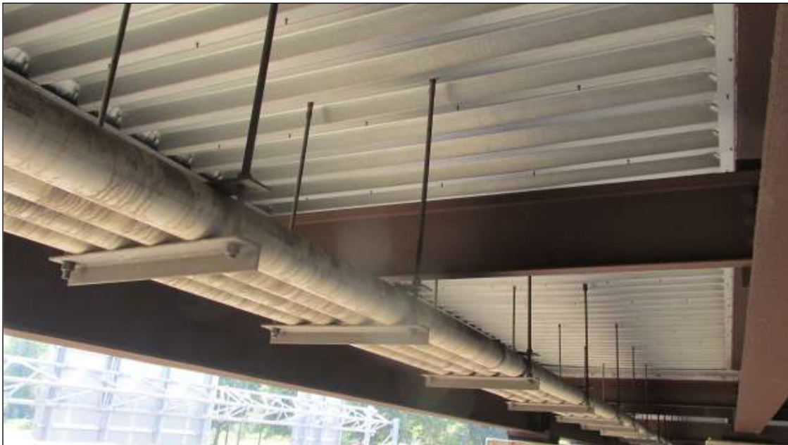
UTILITY UNDER BAY 13
