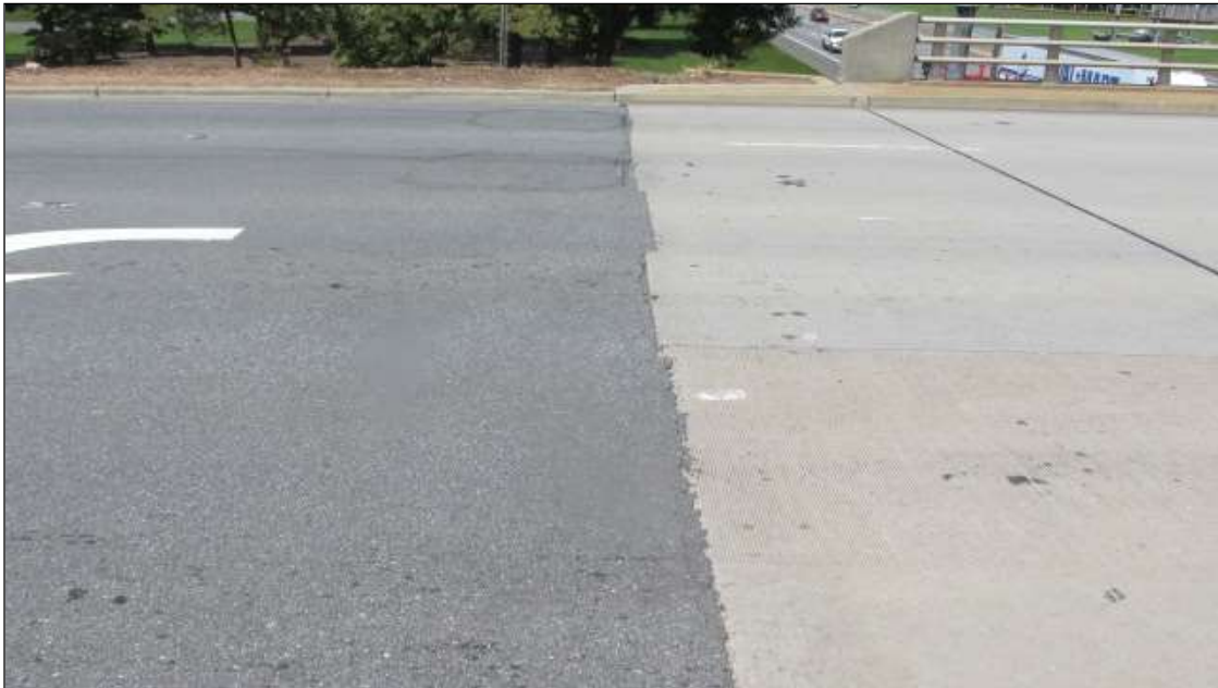
CHIPPING OF ASPHALT ALONG THE FILLFACES AT BOTH APPROACHES.
